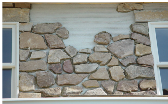
View showing scratch coat, corner & field installation
